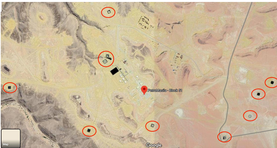
Satellite image of apparent holding ponds, Block 51, Hadramawt.
